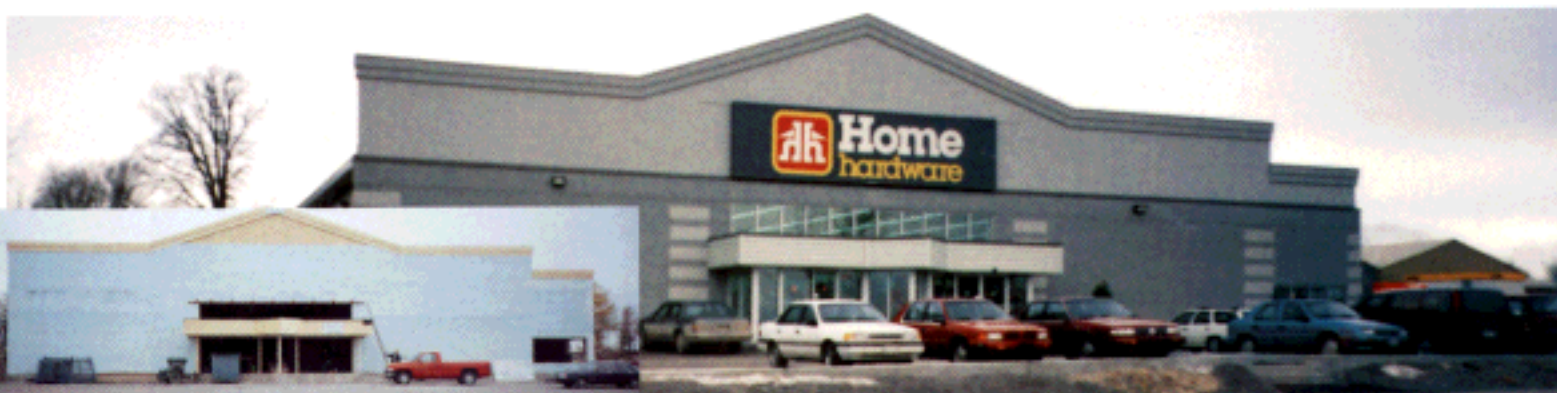
Home Hardware Building - "I am very satisfied. Performance of the building has been excellent, even better than we expected. This is the only way to build... I'm planning another building using ICFs. It is just a great building product." John Lamoureux, Owner
