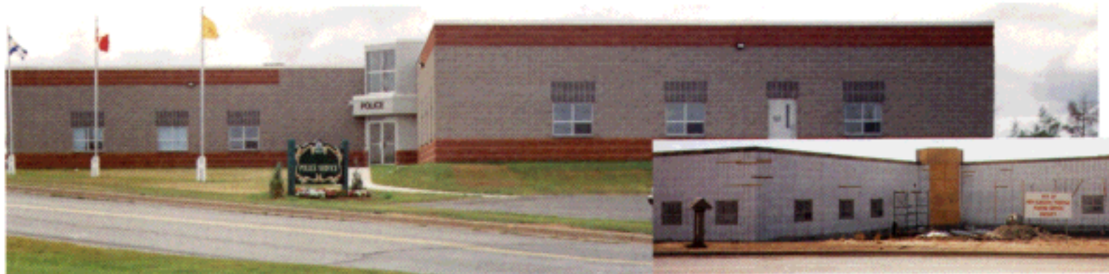
New Glasgow Police Services Building - "Costs for the conventional design of our new police station were well in excess of the $2 million budget. Our project manager submitted a proposal using ICFs. The building gave us improved quality and more amenities. It was better suited to the end use, and was within budget in spite of a winter construction schedule. The town is very pleased with the results." Bob Funke, Town Engineer
